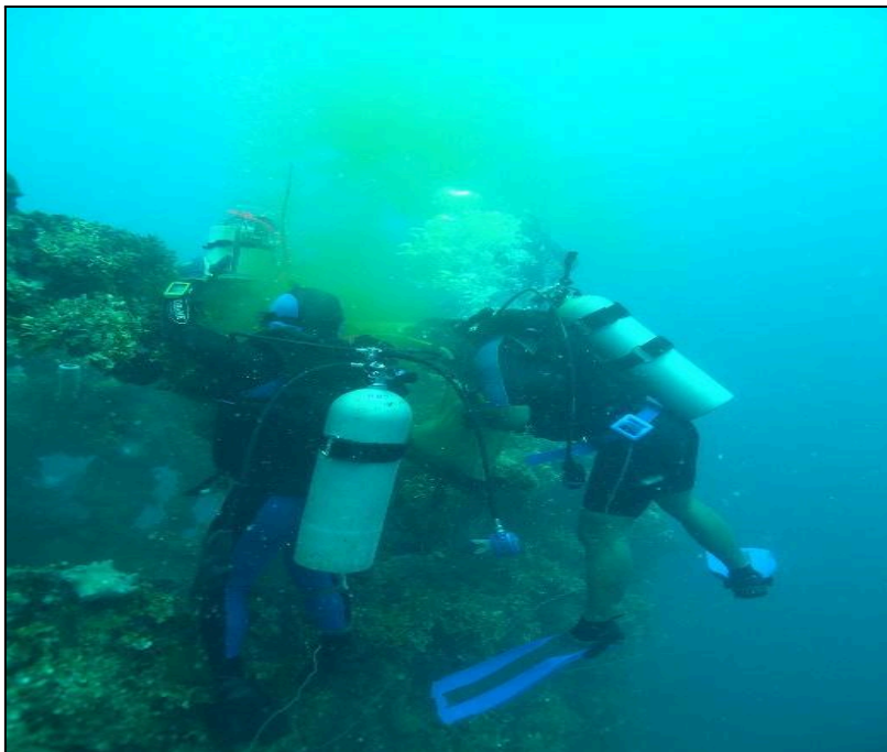
Figure 4: Ian MacLeod and Arimichy Rudolph measuring active corrosion on the Tonoas dock boat. Note the "rust clouds" released during the assessments. Photo by Anerit Mailo 2008.
